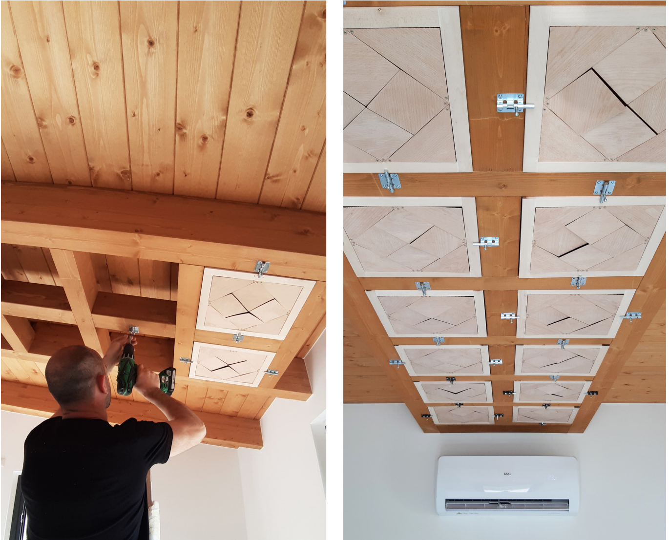
Fig. 6: The “unplywood” panels fixed to the false ceiling.
